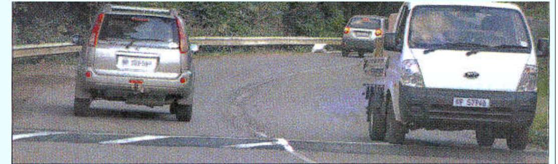
PHOTO: MARK WING The newly installed speed humps just below World's View on Old Howick Road. There are no rumble strips or warning signs for approaching motorists to slow down, but this is about to be fixed.
