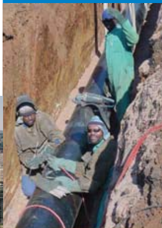
BULK POTABLE STORAGE & DISTRIBUTION
